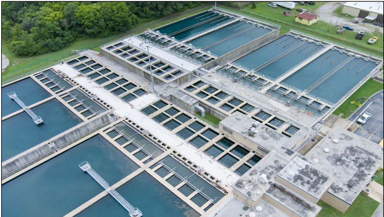
The two photos above show the South Parkway Water Treatment Plant, one of three Huntsville Utilities facilities that treat water taken directly from the Tennessee River. Over $23 million will be spent to rehab this facility which has been in service since 1964. The project is being funded through low interest Alabama State Revolving Fund (SRF) loans and is expected to be complete in 2025.
